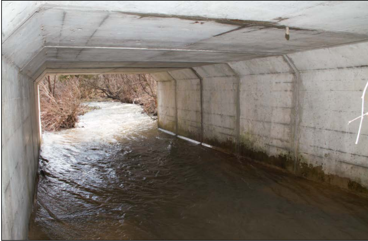
Figure 3. Reach of Shotwell Brook used for velocity and area measurements. The photograph was taken at the overspill, looking upstream.
