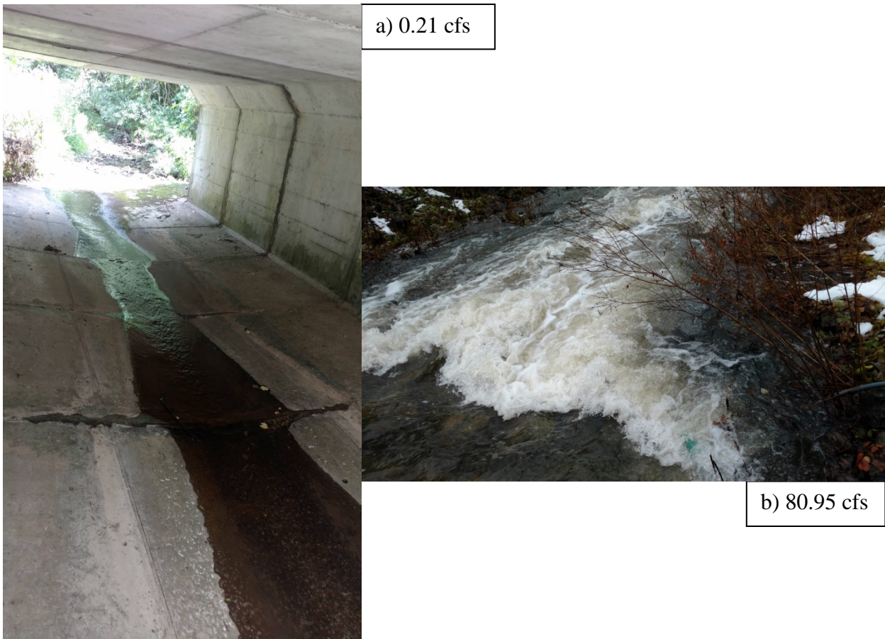
Figure 9. Photographs of Shotwell Brook under the State Route 41 bridge: (a) low streamflow on July 6, 2018 and (b) high streamflow on November 27, 2018.
